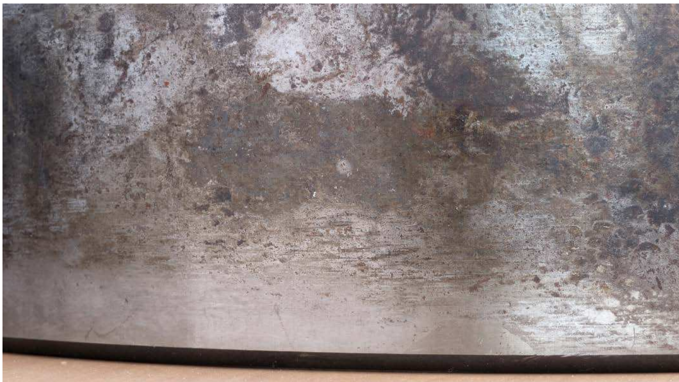
Fretting corrosion on the outside surface of a bearing outer ring due to a damaged raceway
