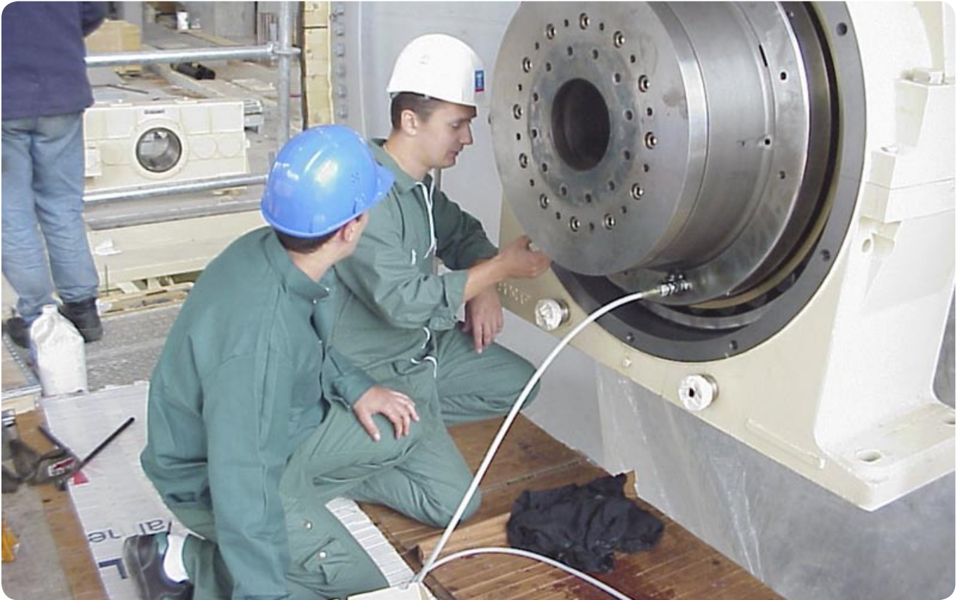
Mounting CARB toroidal roller bearing on a Yankee cylinder using the SKF Drive-up method
