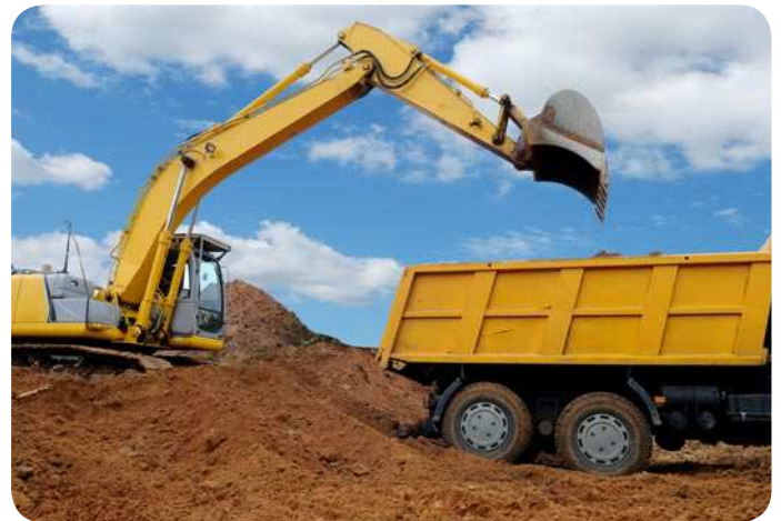
Cabin rotation control and angular position of joints
