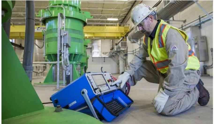
Testing a motor with the AWA-IV 12kV
