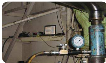
Load cell and hydraulic jack near shaft bearing
