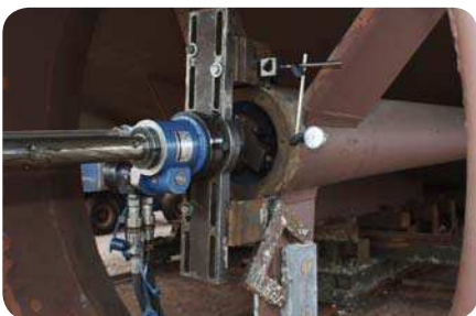
On-site machining of a stern tube
