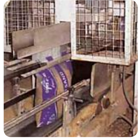
Tarmac Trupak sand bagging facility
