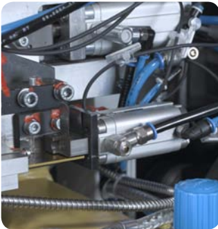
Replacement of pneumatic cylinders
