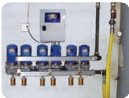
Dryer assembly #640810 is rated for maximum 200 SCFM and includes PLC box (1/4\"/>
