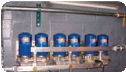
Dryer assembly #640600 is rated for maximum 120 SCFM with standard timer and optional 619785 manifold and mounting kit.
