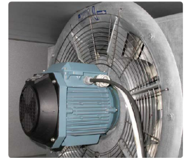
Fan installation at Sunderby Hospital
