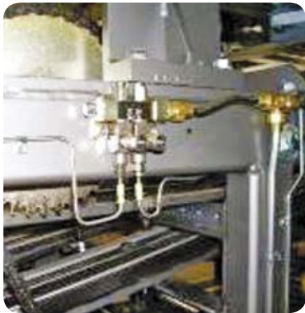
Stainless steel SL-32 grease injectors are used here to prevent corrosion from daily "wash-down" maintenance practices at this food plant.
