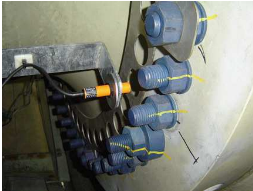
Figure 3-2. Connection of Pulse Transmitter.
