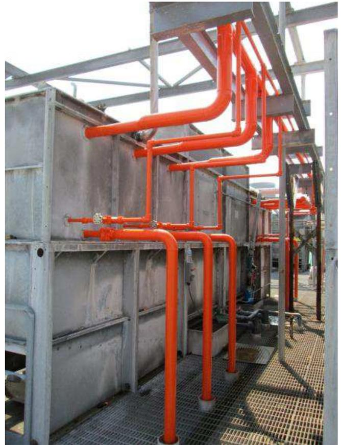
**Corroded pipes identified through frequency inspection allowing for planned project replacement before any failure.**
