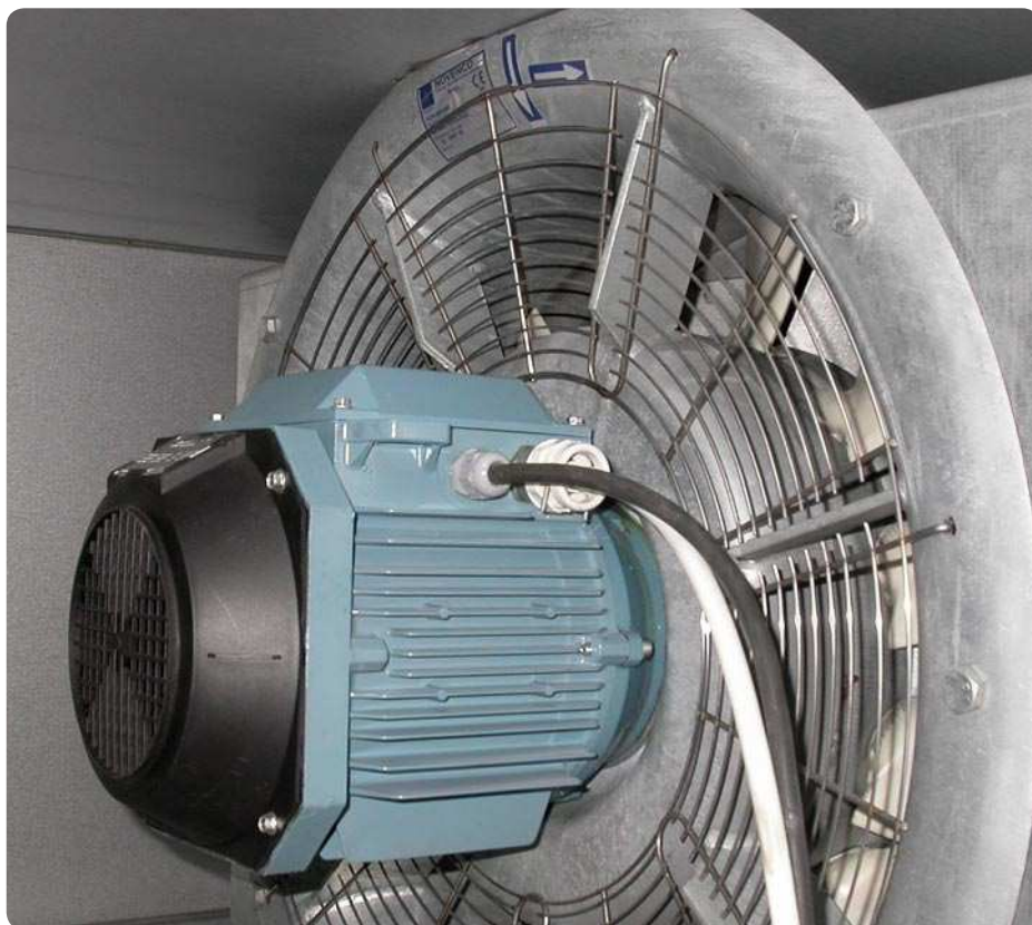
Fan installation at Sunderby hospital
