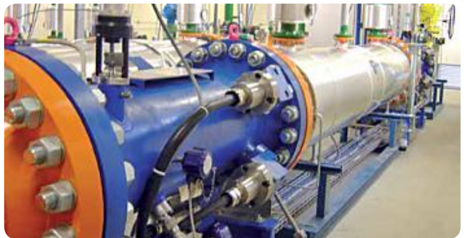
Gas Verbund Mittelland (GVM) natural gas pressure let down recovery station can deliver a total of 600 kW (2 stages).workshop
