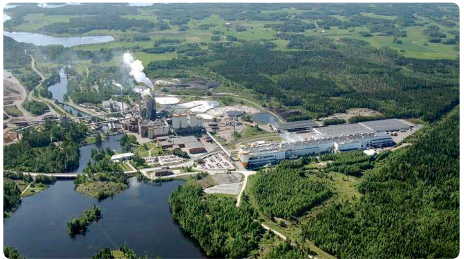
Aerial view of AssiDomän Cartonboard AB in Frövi, Sweden
