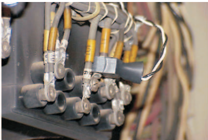
Examples of CT connections to the secondaries of the protection CTs.
