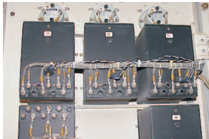
Examples of CT connections to the secondaries of the protection CTs.
