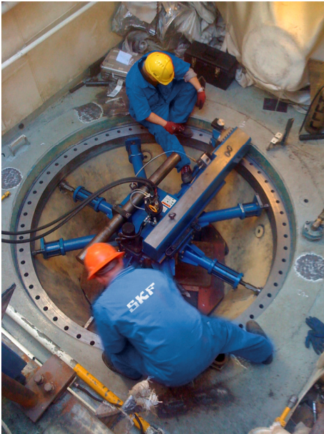
Caption: SKF service engineers perform on-site machining of a flange face.
