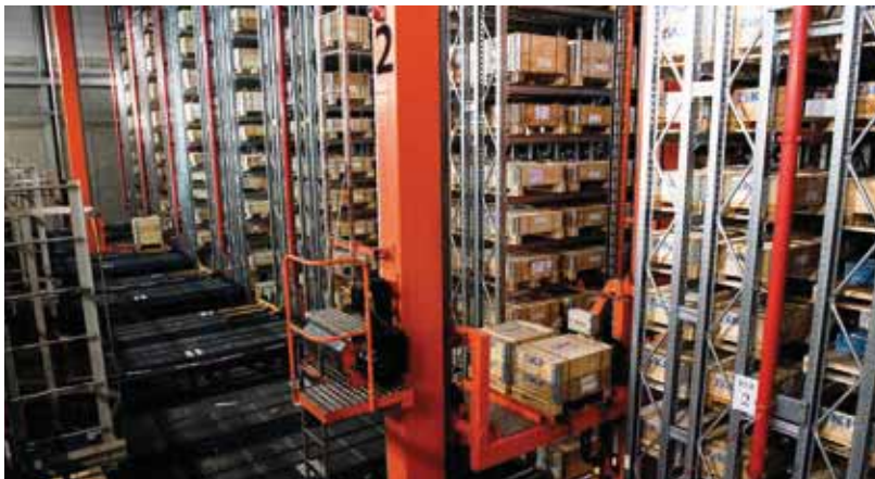
The European Distribution Centre in Belgium has further increased its capacity for the Mini-Load system, a highly efficient and automated goods retrieval system with quadrupled productivity.
