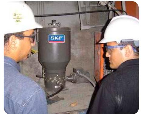
The SKF system also reduced the facility's lubricant consumption, cutting it from an average of 100 kg of grease per week to 35 kg, for a monthly savings of nearly \$1 000. The system also enabled the facility's maintenance team to begin focusing on other duties, and kept them safely away from hot clinker cooler particles.
