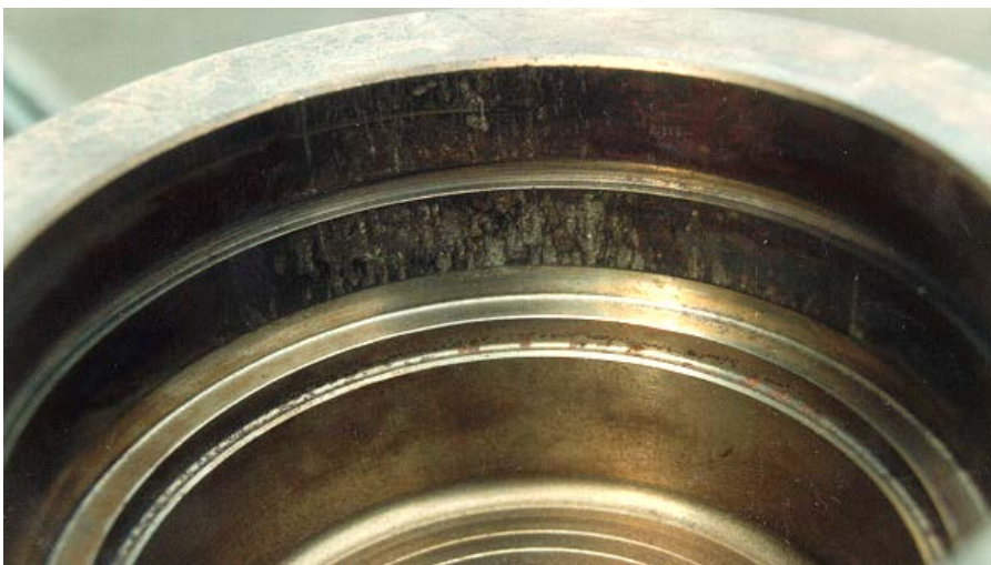
Fig. 7 Fretting corrosion in the housing
